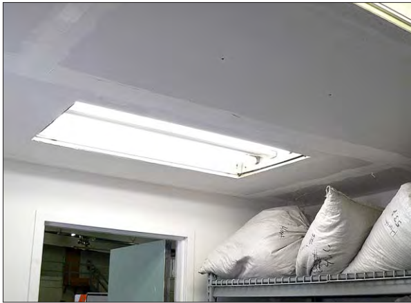
A screened enclosure and a mudded, drywall ceiling (left) protect seed from rodents. Window and wall air conditioners and dehumidifiers create climate-controlled conditions (right).
