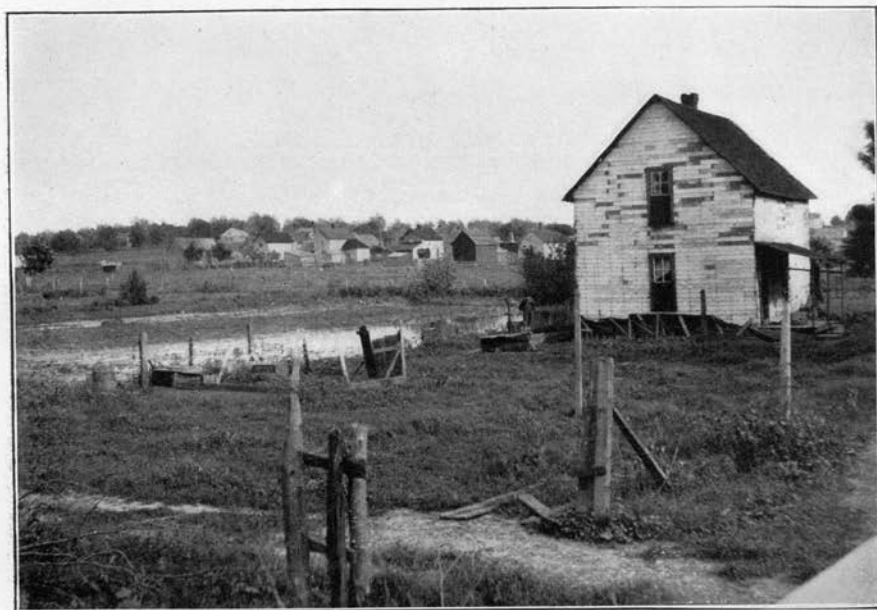
Fig. a. A pond and well in Marshalltown, showing the location of the well close by the pond. Bad surface water.
