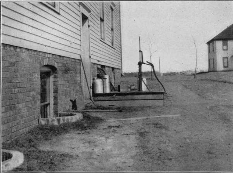
Fig. a. A Colonial club-house well. Well with excellent surroundings, neat and clean, on a hill; the well over 100 feet deep and yet containing a large number of organisms. Probably an underground channel occurs, or perhaps there is a leak in the pipes.
