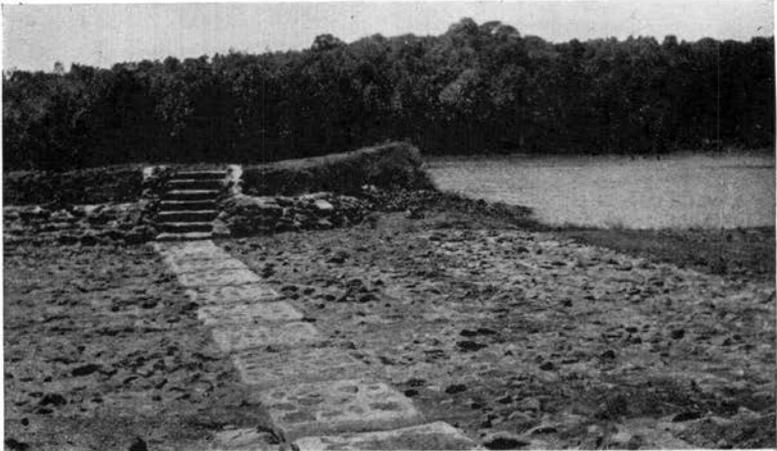
Fig. 6. Silt dam spillway
