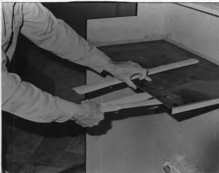
Figure 15. Using Supports to Align the Laminate over the Substrate
