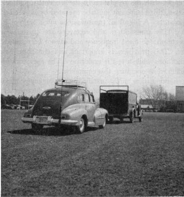
Figure II. The test car and control car showing radio control and communication antennas.
