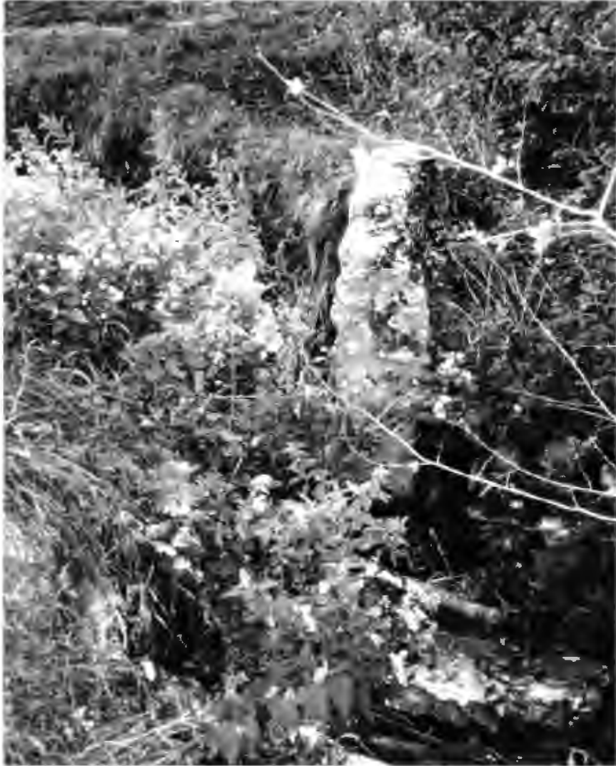
Figure 10. The north end of Dam 1. The location of the old gully bank from when the dam was built can be seen about three-quarters of the way down the center of the photo where the main wall starts to slant inward. The remnant of the extension of the side wall that fell down in the gully as it formed around the dam can be seen to the lower right of the photo.
