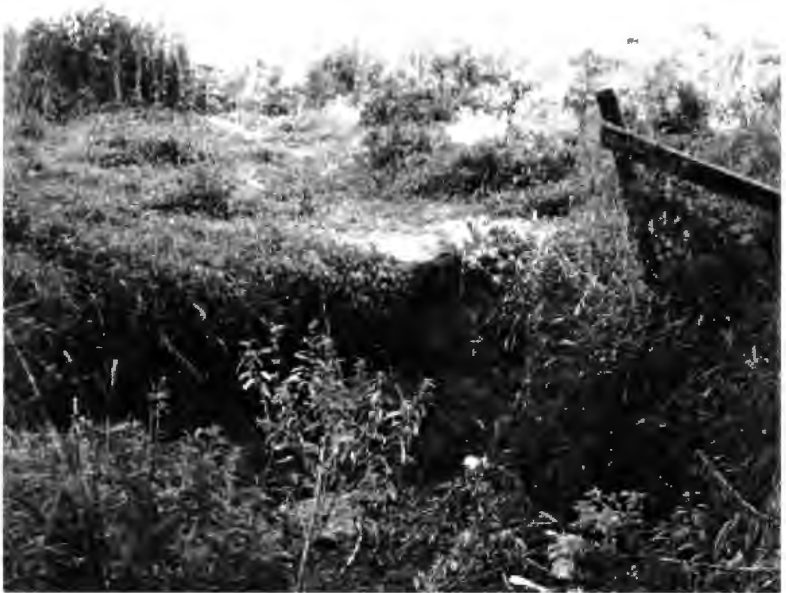
Figure 15. Headscarp upstream of Dam 1.
