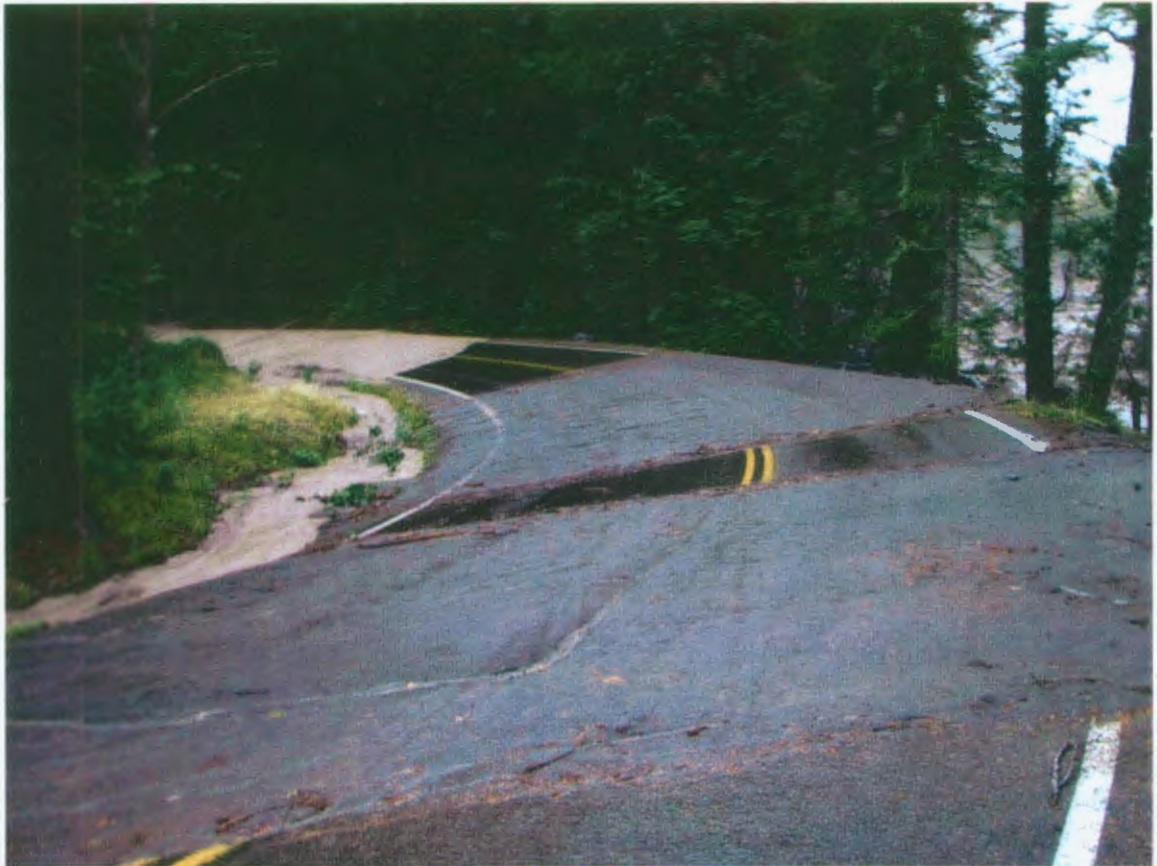
▲ FIGURE 6.3 Van Trump Creek flowing across Lower Van Trump Hairpin during the fall 2005 debris flow. (Photo: National Park Service, 9/29/2005)
