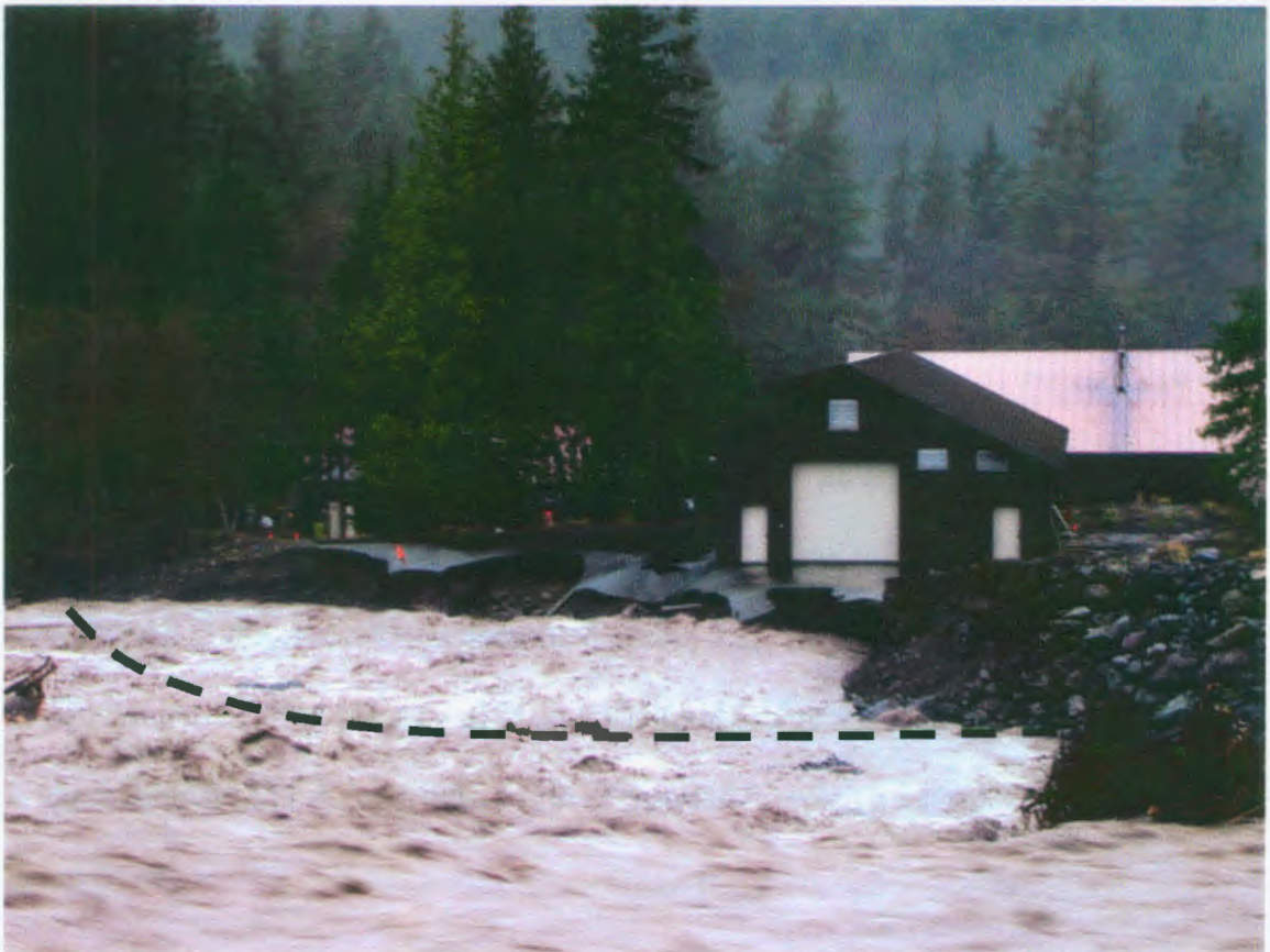
▲ FIGURE 5.1 Damage to Emergency Operations Center, levee and parking lot from flooding in November 2006. Dashed line shows approximate former levee boundary. (Photo: National Park Service, 11/17/2006).
