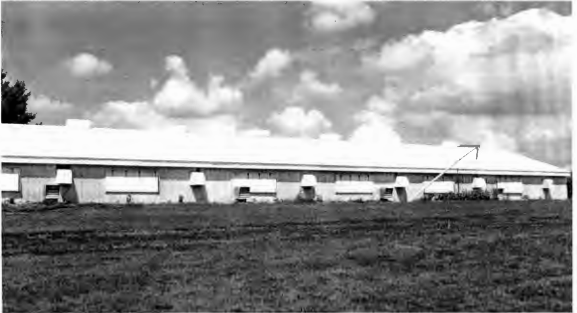
Fig. 7. Mechanically ventilated confinement. Note the presence of six sidewall fans and four pit fans.
