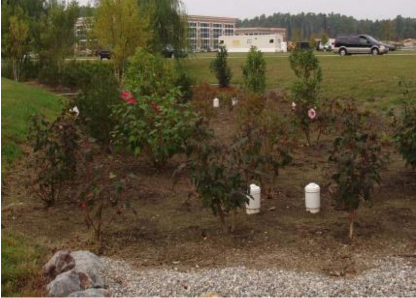
Figure 2: A bioretention cell located in a Williamsburg, Virginia parking lot. Photo included in a workshop flyer developed by Virginia PRIDE Water Quality Education Program.
