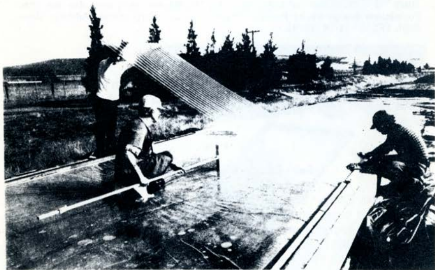
Fig. 3. Experimental shallow solar pond under construction at Livermore. The pond is one-quarter the length of a normal module, but it provides enough information on incident solar radiation and heat collection to permit extensive calculations.
