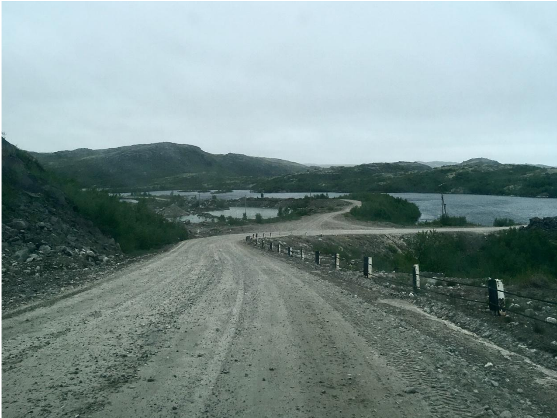
Figure 2. The unpaved section of the road from Murmansk to Teriberka. July 12, 2019.
