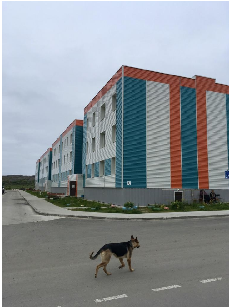
Figure 16. The renovated residential building in Lodeynoe (Teriberka). July 15, 2019.
