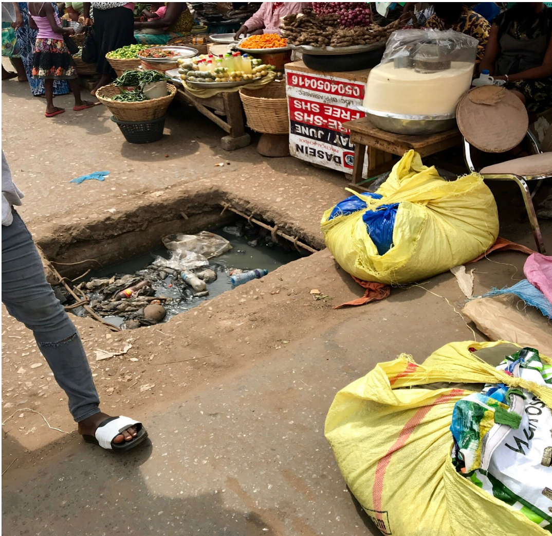
Figure 2 Choked Drain at the Ashaiman Market
