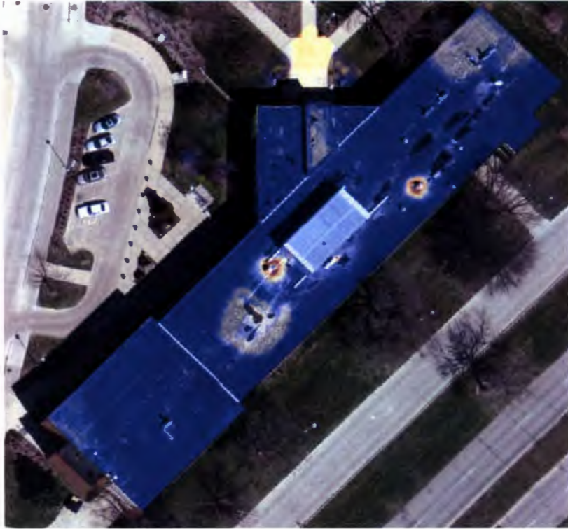
Figure 15. Thermal data overlay, Latham Hall.
