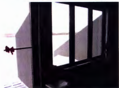
Of interest in this photograph are the wing walls. Designed to reduce low sun angles from entering the building, one can also see how they help to create separate viewing areas, increasing privacy.
