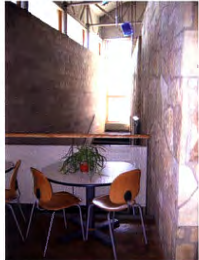
This image was taken on the upper level of the CEEE looking West. Notice the Maquoketa limestone wall on the right and, concrete block on the left. Tall, but narrow west window at the top of the staircase, illuminates the entire length of the staircase with the help of the clerestory windows along the south wall.
