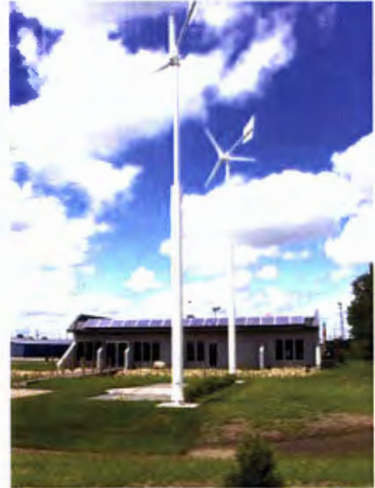
This image shows the wind turbines as well as the photovoltaic panels on the roof.
