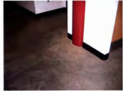
This image shows the concrete flooring and the surrounding wall finishes.
