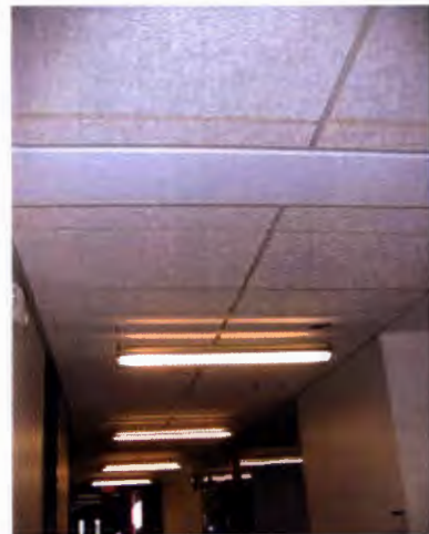
Acoustical tile panels are found almost everywhere, however, few have seen the wheat board acoustical tile panels. Similar to their traditional counterparts, these panels serve to absorb the sounds that a concrete floor and flat painted walls of a hallway can produce. At the same time they add a unique texture to the ceiling.
