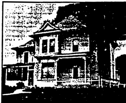
Poweshiek County Historical & Genealogical Building
