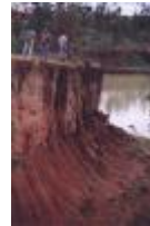
The edge of a previously mined area.
