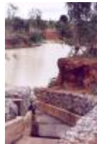
Heipang gullies provide drainage into previously mined areas.
