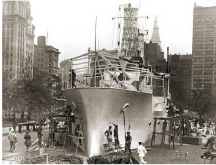
Fig. 07: In 1918, the U.S. Navy built a temporary wooden recruiting station in the middle of Union Square in New York City. Shaped like a ship in every detail, it was christened the USS Recruit. In July, as a way of calling attention to recruiting and fundraising, the Women's Reserve Camouflage Corps painted the landlocked vessel in a riotous "dazzle camouflage" scheme. The camouflage plan was developed by men.
