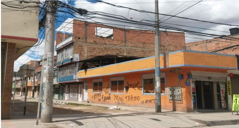
Figure 29. Brick houses in Bosa (photo by Ekaterina Korzh).
