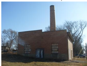
Figure 1. Boiler house and smokestack on 13 th Street, Cedar Falls, IA.
