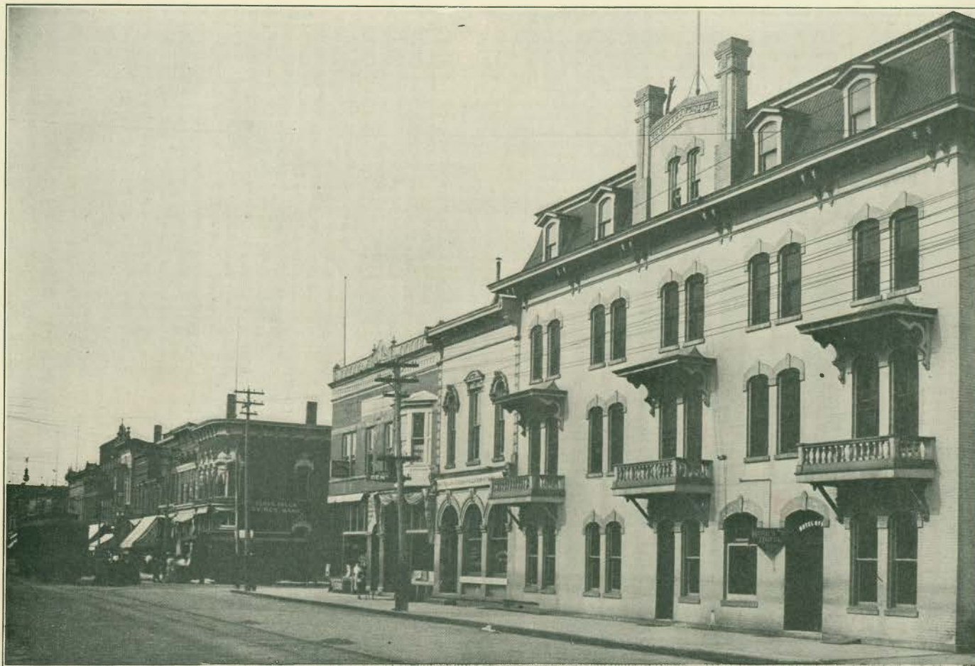
MAIN STREET, CEDAR FALLS, LOOKING SOUTH.
