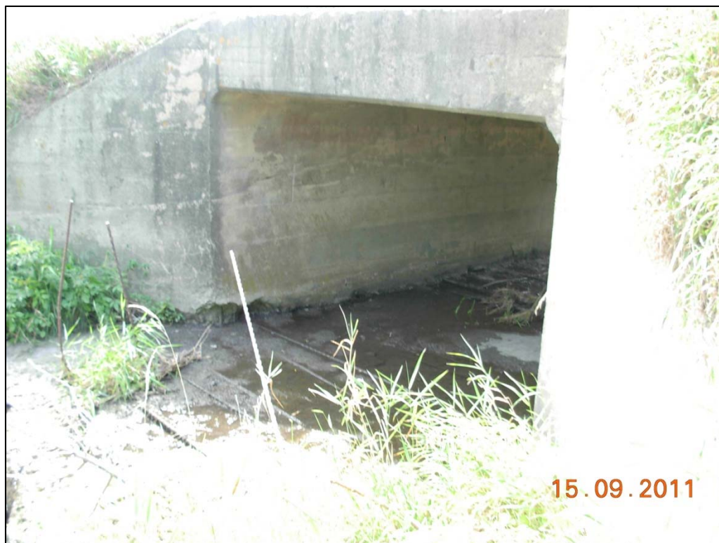
Figure 9. Photo of Site 4.
