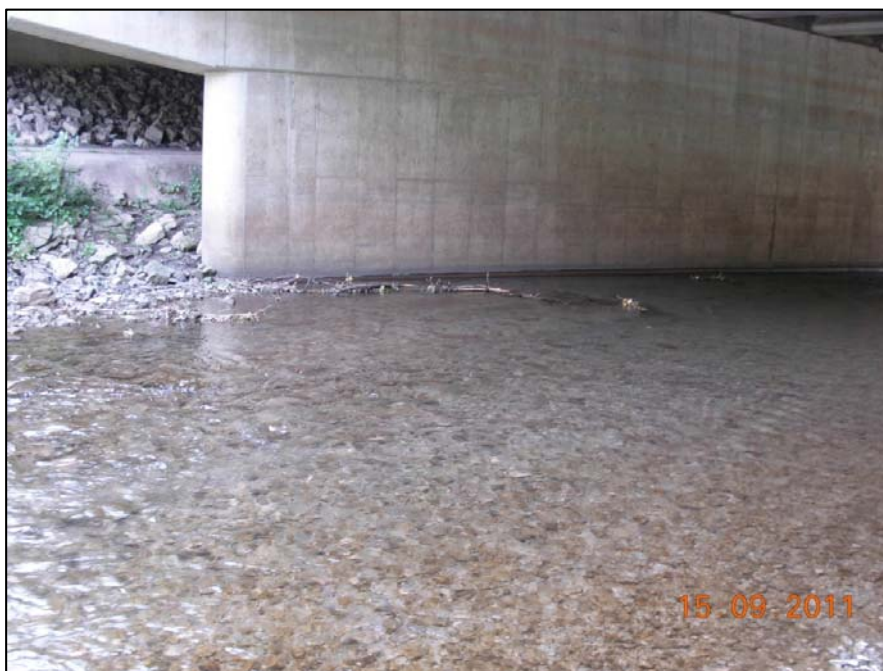
Figure 13. Photo of Site 8.
