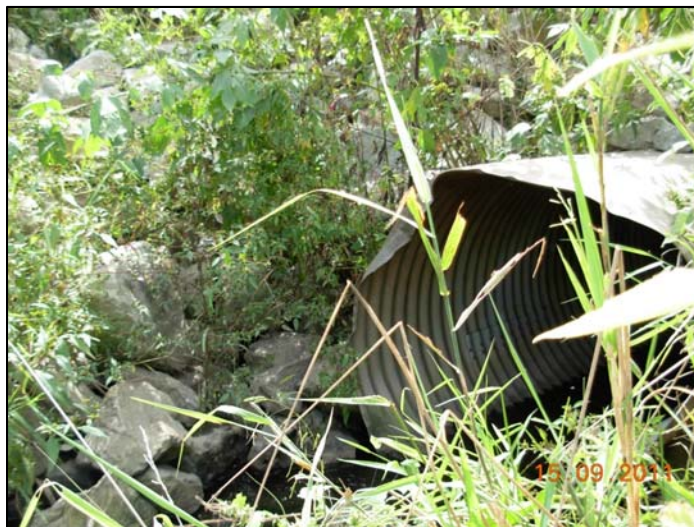
Figure 14. Photo of Site 10.
