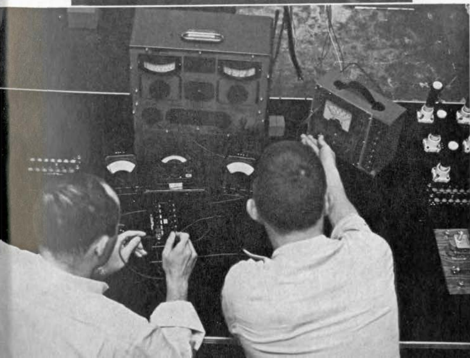
Testing Electrical Equipment
