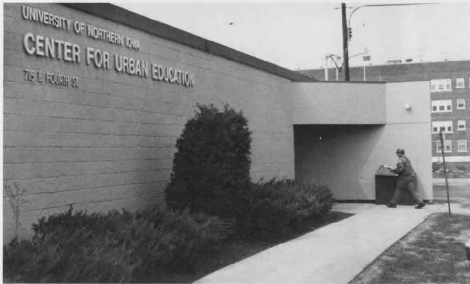
UNI-CUE operates in Waterloo, twenty minutes away from campus. The building's costs and maintenance are funded jointly by the university and the federal government. Photo by David Wagner.
