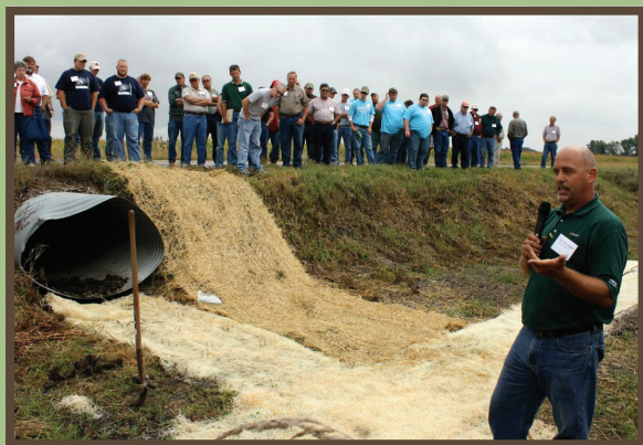
Steve Krehbiel of Quick Supply Co. demonstrating erosion control materials for the Roadside Conference bus tour.
