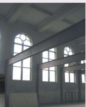
**Kudos to** those continuing the progress of Sabin Hall! *Above:* The old lecture hall has been fitted with beams to support a new floor of space for faculty offices. *Left:* The new lecture hall, moved one floor below its old location, takes shape. The tiered seating will be oriented toward the windows, which face the Union and will be fitted with movable panels to create the projection surface.
