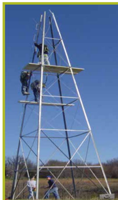
Industrial Technology students construct a wind tower at Hickory Hills Park.
