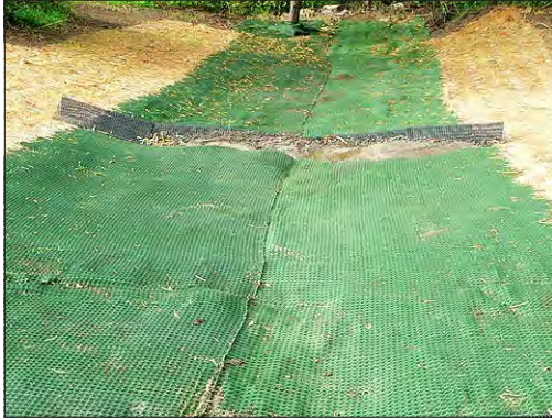
Left: TRM in use with ECB and ditch check to provide both erosion and sediment control. Right: A lightweight TRM (green) is used where a moderate-flow channel becomes steep, while a heavyweight TRM (brown) protects against very high flow from a 36 in. culvert.
