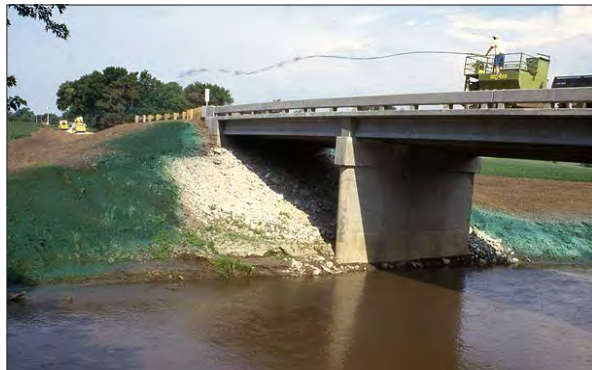
Top right: Ditch cleanouts can leave a steep foreslope. By angling the gun and using a concentrated stream, seed will be embedded in the slope. Bottom right: Hydroseeders can be very useful for challenging sites. Bottom left: Using a loader tractor to load mulch bales saves time and backs.
