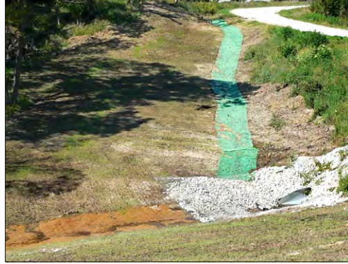
Left: TRM in use with ECB and ditch check to provide both erosion and sediment control. Right: A lightweight TRM (green) is used where a moderate-flow channel becomes steep, while a heavyweight TRM (brown) protects against very high flow from a 36 in. culvert.
