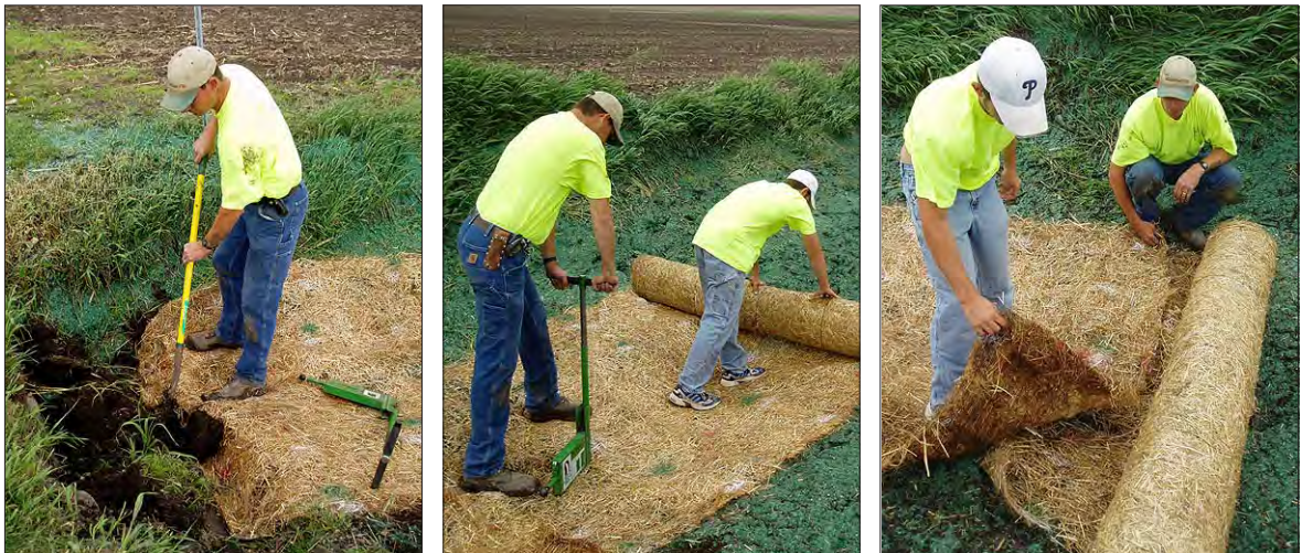
When installing ECBs, trench the top of the blanket 6 in. and staple at the bottom of the trench. Follow manufacturer specs for stapling patterns. Tuck the downstream blanket at least 6 in. under the upstream blanket to prevent flow from getting under the blanket.
