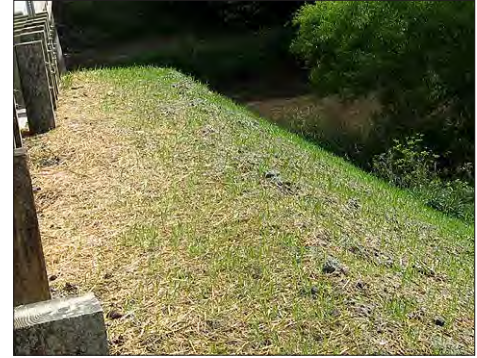
An innovative 3-step method was used on this critical slope: 1) hydroseed with tack and paper mulch, 2) blow on straw, 3) hydromulch with more tack and paper mulch to “stick” the straw and seed.
