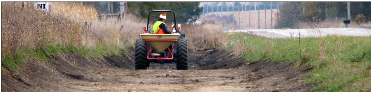
Broadcast seeding in mid-fall following a ditch cleanout.
