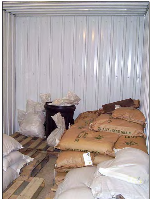
This seed room is “sealed” with tin to keep out rodents and provide a moisture barrier.
