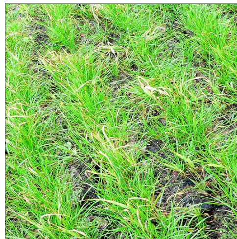
Pulling a ripper perpendicular to the slope creates grooves that slow runoff. When followed by hydroseeding, vegetation germinates and grows in the grooves, creating a drill-row appearance.
